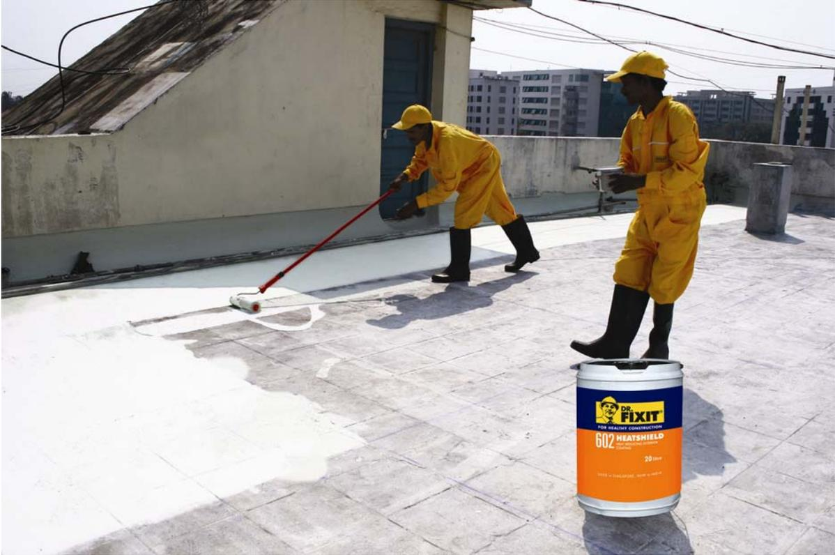
Figure8. Application of heatshield on a concrete surface
