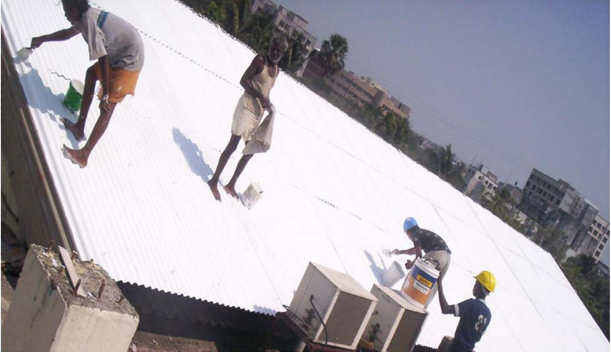
Figure9. Application of heatshield on a metal surface
