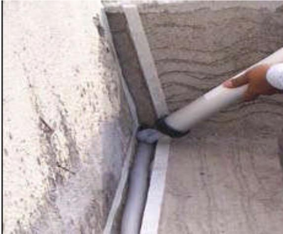
**Fig: 3 Application of PU sealant**
