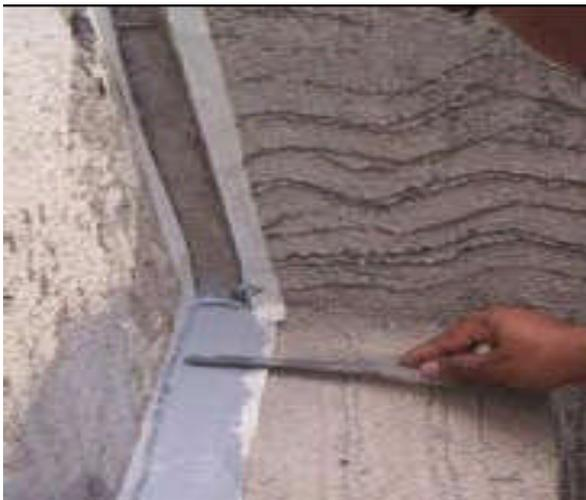
**Fig: 4 Tooling of excess sealant**
