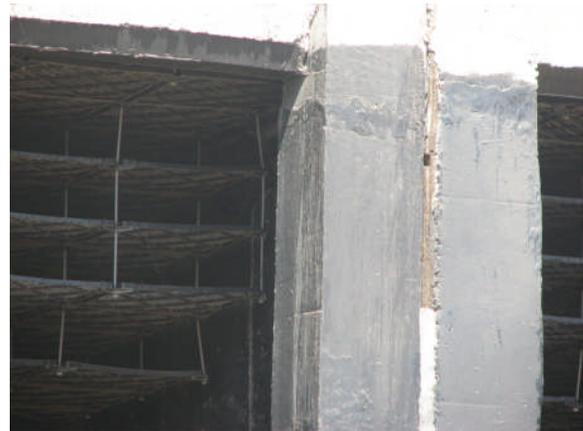
**Fig: 2 PU sealant at construction joint**
