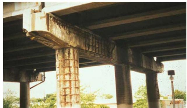
Fig. 2. Corrosion of steel reinforcement due to carbonation in a bridge
