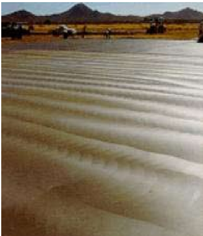
Figure 5 : Application of SRA Concrete
