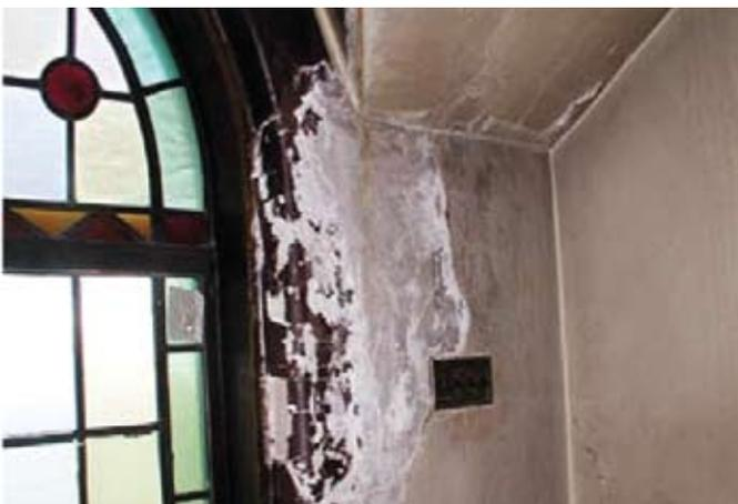
Fig 2: Distress in plastering
