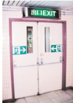
Fig. 2: Emergency exit door
