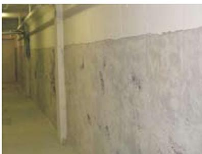
Fig. 1: Surface prepared for application of crystalline coating
