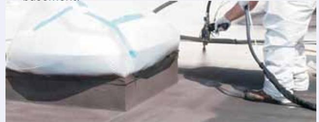
Fig. 14: Spraying of Hybrid Rubber Neoprene system
