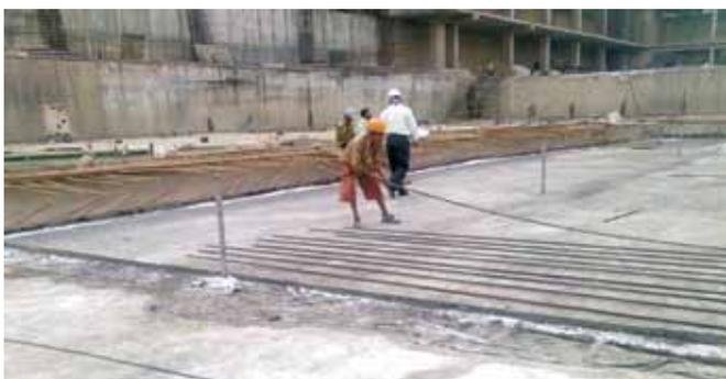
Fig. 12: Installation of EPDM based membrane system
