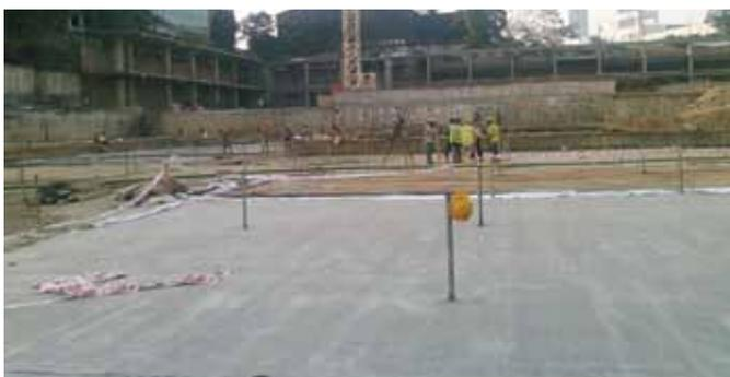
Fig. 13: View of EPDM based waterproofing membrane system
