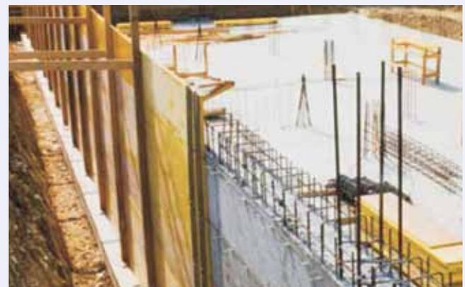
Fig. 9: SBS sheet membrane applied in double layer to concrete foundation wall in a basement
