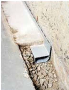
**Fig. 7:** Installation of footing drain pipe at wall and floor junction
