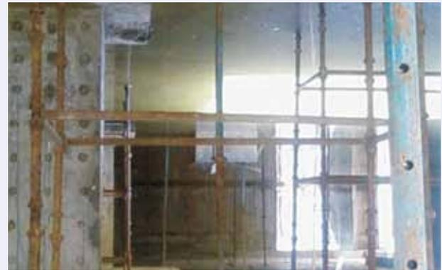
**Fig. 4:** Grouting of basement wall
