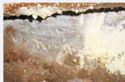
Fig. 3: PU forming foam after the injection
