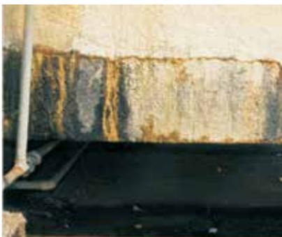
Fig. 1: Leakage in a roof terrace water tank
