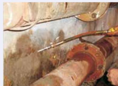
Fig. 2: PU injection in a water retaining structure
