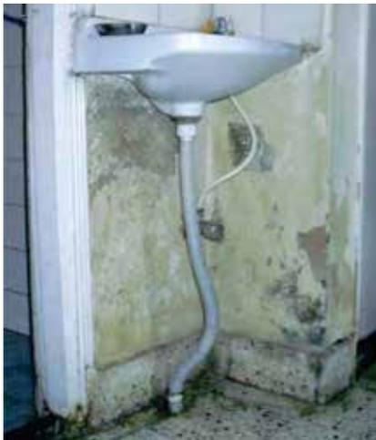
Fig. 3: Dampness around a wash basin causing the paint of the wall to peel
