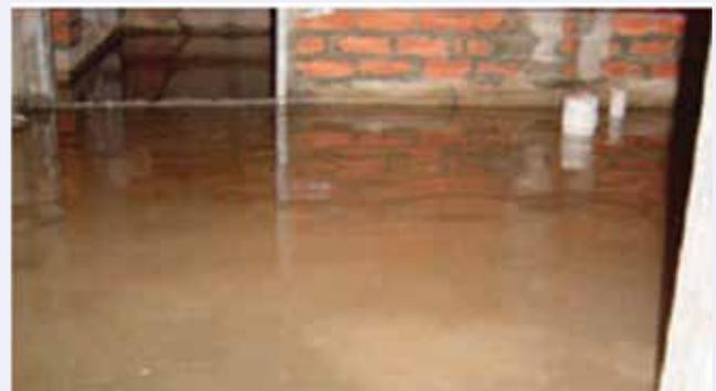
Fig. 26: Water ponding in bare concrete slab of bath room
