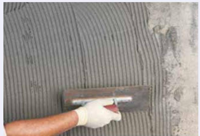
Fig. 29: Fixing the tiles with tile adhesive
