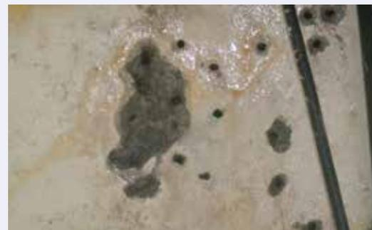
Fig. 2: Water dripping and accumulation on the surface of a roof slab
