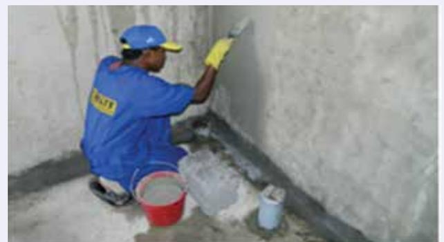
Fig. 24: Application of 1st coat cementitious coating on wall
