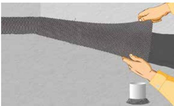
Fig. 21: Laying of glass fibre mesh
