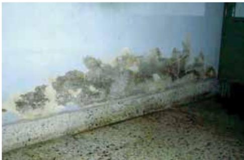
**Fig. 4:** Capillary rise of water causing efflorescence
