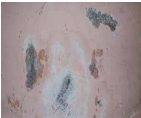
**Fig. 5:** Stains and blistering of paint in kitchen
