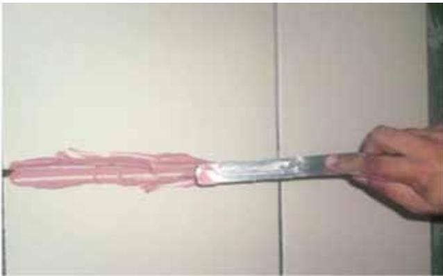
Fig. 30: Filling the joints with tile grouts
