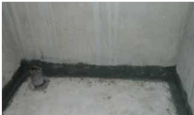
Fig. 20: Providing angular fillet around the periphery of wall
