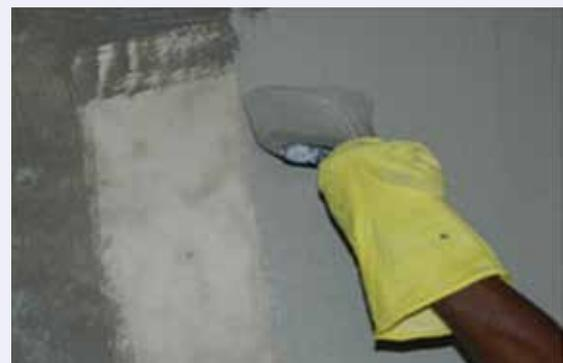
Fig. 23: Cementitious coating on floor
