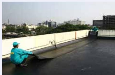
b. Aligning the torch shield membrane
