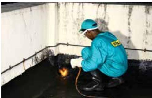
g. Torch-on for fixing at termination end of parapet
