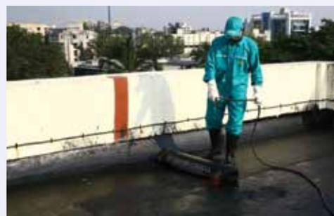
c. Torching the membrane by acetylene gas and pressing hard on the surface
