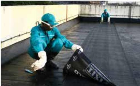
e. Aligning the adjacent roll with an overlap of 100mm
