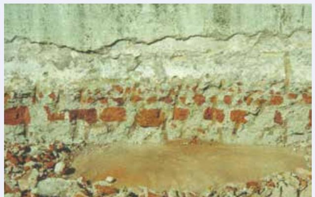
Fig. 6: Three layers of Brick-bat-coba increasing the dead load on the structure
