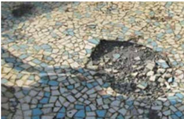
Fig. 7: Cracks developed in China mosaic waterproofing system
