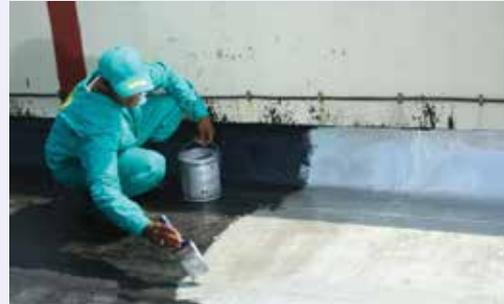
h. Finishing with aluminium coat for non-foot traffic or else screeding for foot traffic
