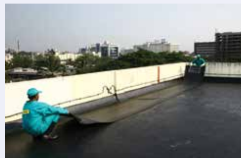
b. Aligning the torch shield membrane
