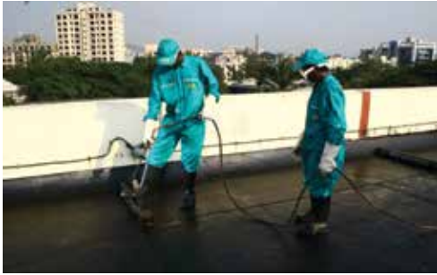
d. Simultaneously doing the torch-on and pressing the membrane
