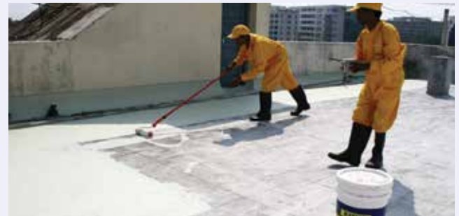
b. Applying the 1st coat
