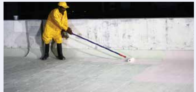
c. Applying the 2nd coat
