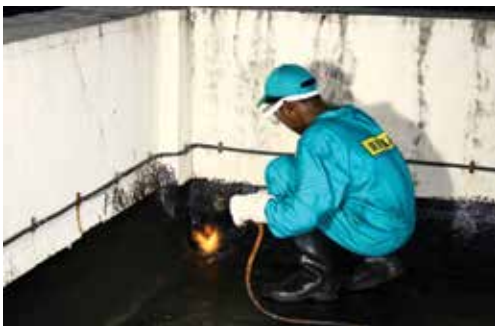
g. Torch-on for fixing at termination end of parapet
