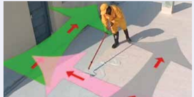
d. Applying the 3rd coat perpendicular to 2nd coat
