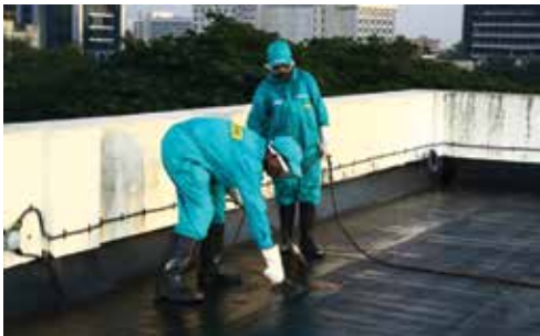
f. Torch-on at the overlap portion at the joint
