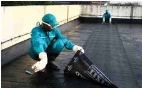
e. Aligning the adjacent roll with an overlap of 100mm
