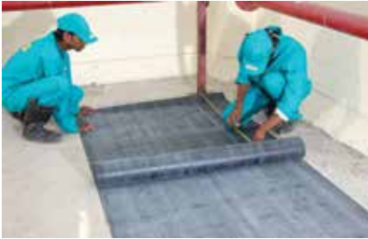
Fig. 16g: Taking the measurement for a cut piece member
