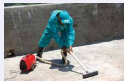
Fig. 16b: Mechanical cleaning of the surface
