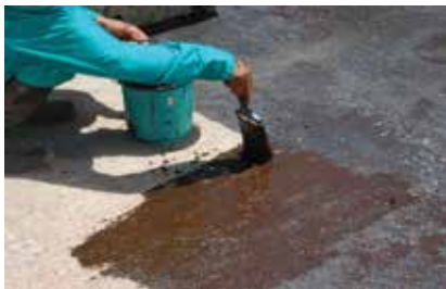
Fig. 16d: Application of bonding adhesive
