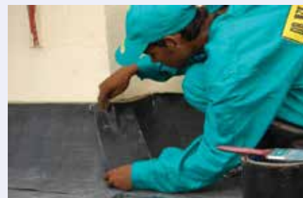
Fig. 16n: Fixing the cut piece membrane at the corner junction
