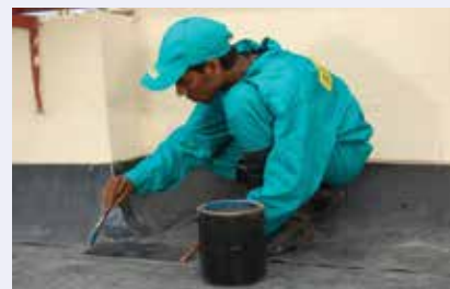
Fig. 16m: Applying the bonding adhesive on back of splice membrane
