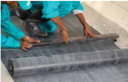
Fig. 16h: Cutting into smaller piece of the membrane
