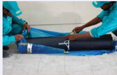
Fig. 16e: Opening the membrane from sealed cover
