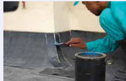
Fig. 16l: Applying the bonding adhesive for fixing the cut piece membrane
