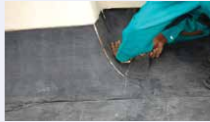
Fig. 16j: Fixing the cut piece at termination end
