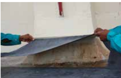
Fig. 16i: Aligning and laying the cut piece membrane
