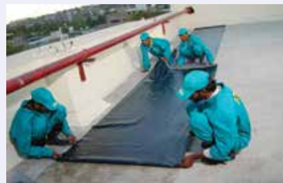
Fig. 16f: Aligning and laying the membrane over primed surface
