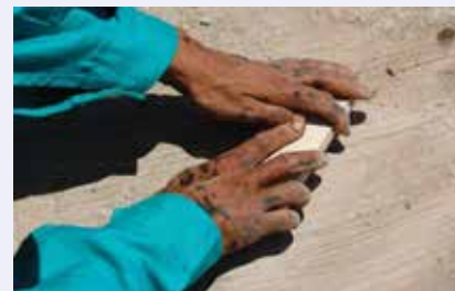
Fig. 16a: Rubbing the surface by wire brush for surface preparation
