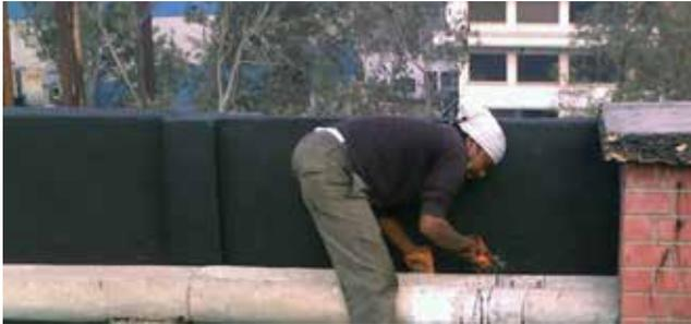
**Fig. 8:** Application of primer in progress
