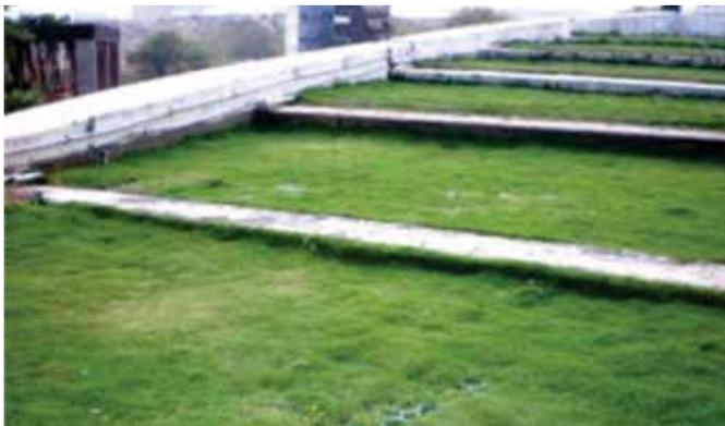
**Fig. 5:** Above figure reveals a section of structural pavers where the sod is thinned, likely a seam
