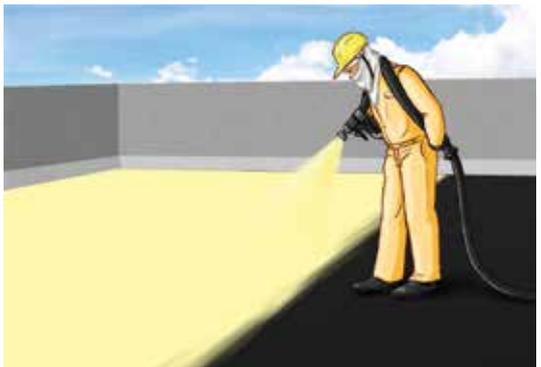
d. Application of spray applied PU foam insulation
