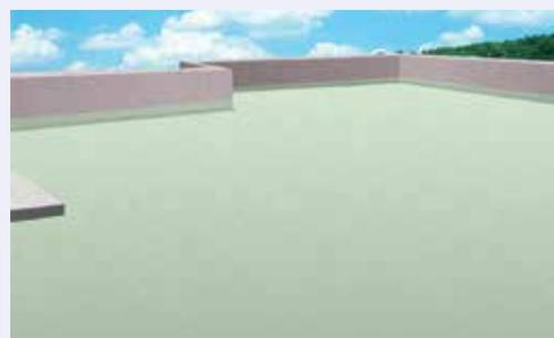
h. Completed Roof With Heavy duty acrylic based waterproofing coating/ highly reflective coating
