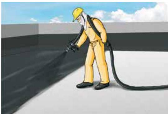
c. Application of spray applied water proofing coating
