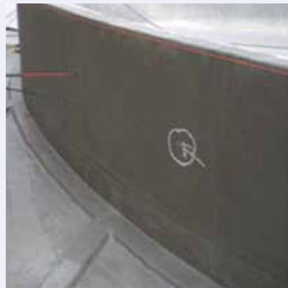
Fig. 12: Remedial waterproofing at leakage point
