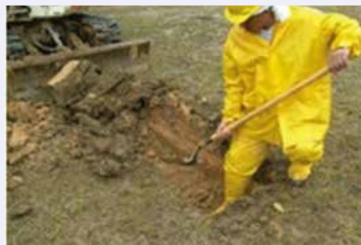
Fig. 8: Pinpointing the leakage location and further removal of overburden for remedial treatment
