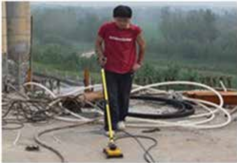
Fig. 8: GPR survey for locating embedded electrical conduits in concrete
