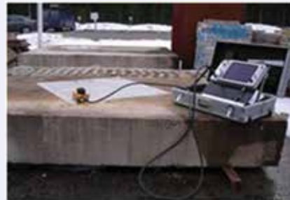
Fig. 11: GPR survey being used to evaluate the deterioration of RCC slab
