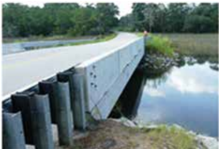
Fig. 13: GPR survey can be used to evaluate the condition of bridge deck
