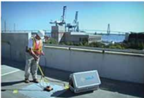
Fig. 9: GPR survey for detecting voids inside concrete
