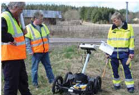
Fig. 4: GPR survey for detecting underground storage tank
