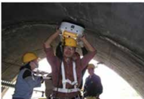
Fig. 5: GPR survey for detecting defects in a tunnel
