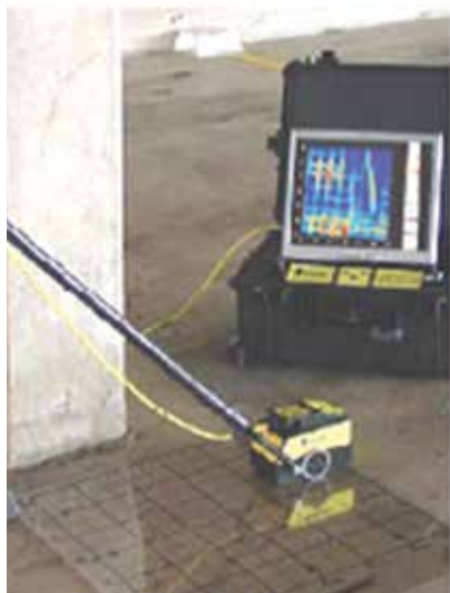
Fig. 2: A GPR survey for concrete structures
