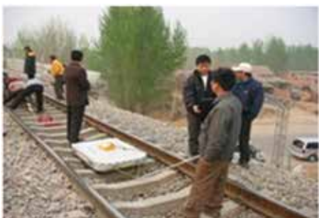
Fig. 14: GPR survey being used to evaluate the railway ballast
