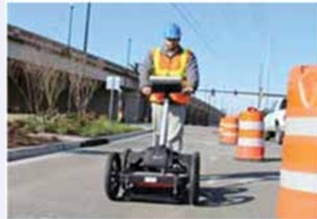
Fig. 1: GPR survey for locating utility services on a road
