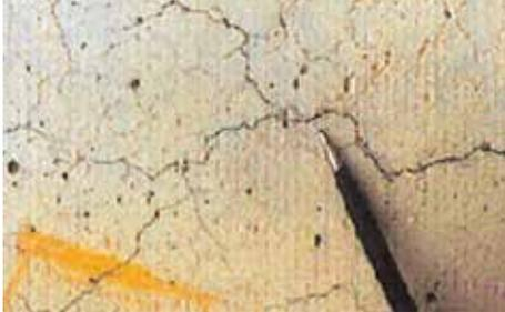
Fig. 4: Map pattern cracking due to ASR
