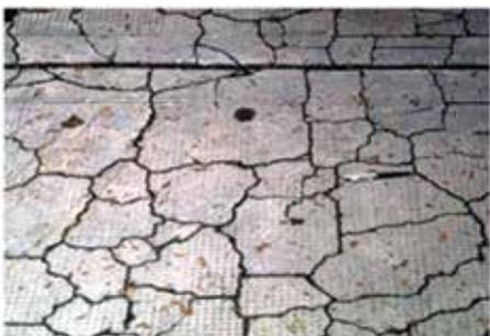
Fig. 11: Map cracking pattern caused by ACR
