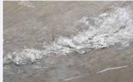
Fig. 5: Efflorescence due to ASR patterns
