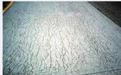
Fig. 2: Longitudinal cracks induced by ASR in a pavement
