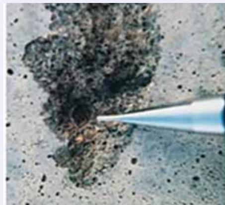
Fig. 6: Popouts due to ASR
