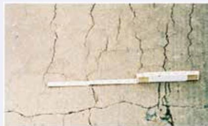
Fig. 3: Close-up view of well developed cracking in a pavement, a typical pattern associated with ASR.
