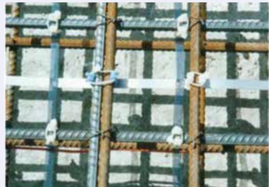
Fig. 5: Ribon anodes being used for Cathodic protection
