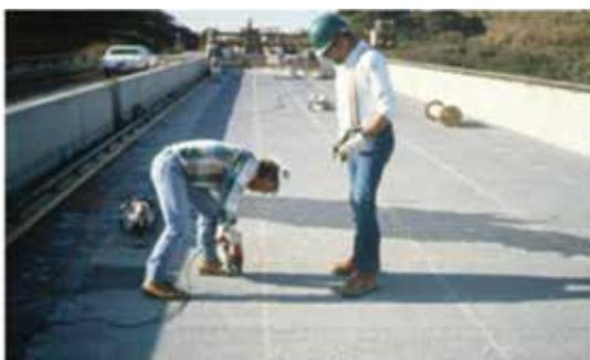
Fig. 2: Anode Mesh installation on a bridge deck
