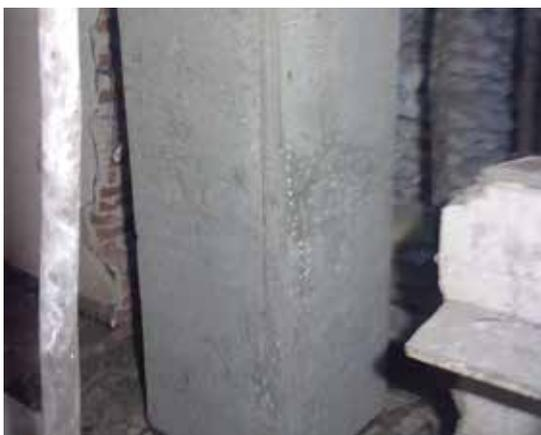
Fig. 5: Column after micro concreting
