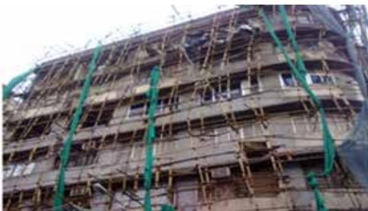
Fig. 1: Continuous sunshade being provided after breaking damaged parties
