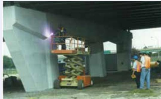
Fig. 3: Arc-spray application of sacrificial Aluminum-Zinc-Indium
