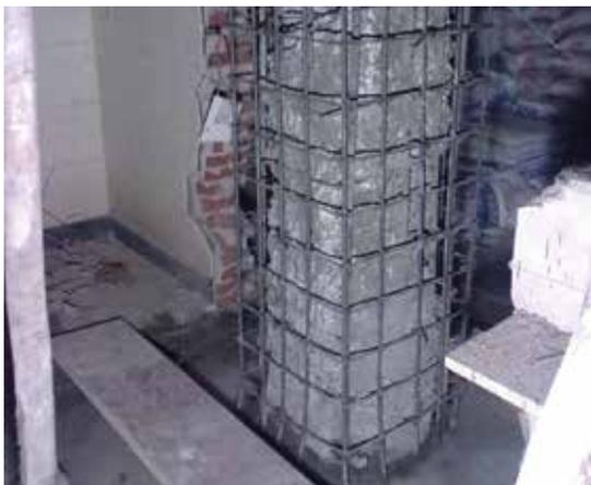
Fig. 4: Column before micro concreting
