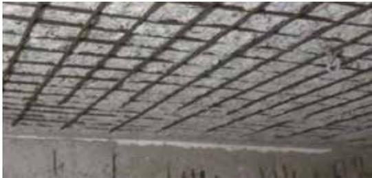
Fig. 2: View of roof slab before micro concreting
