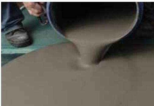
Fig. 1: View of self-levelling cementitious flooring product
