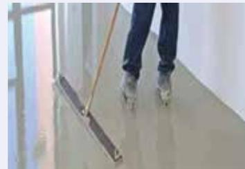
Fig. 2: Spreading self-levelling cementitious flooring product
