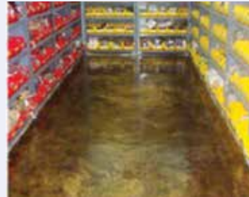
Fig. 21: Floor of Hoovers spares-blast proof machine room before
