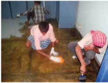
Fig. 16: Priming of floor surface
