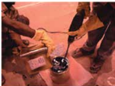
Fig. 3: Mixing of two component primer Dr. Fixit Pidipoxy EP
