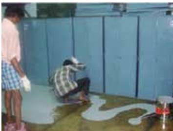
Fig. 18: Application of Dr. Fixit Pidipoxy EP
