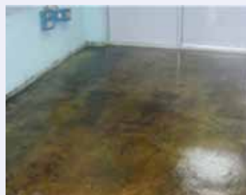
Fig. 23: Floor of TSS Confidential room before
