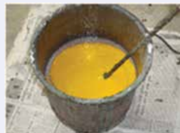
Fig. 8: Mixing of Dr. Fixit Pidipoxy ESL 1000
