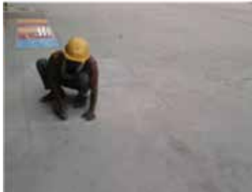
Fig. 1: Inspection of condition of floor
