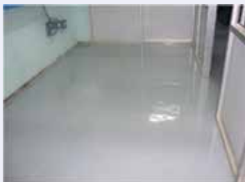
Fig. 24: Floor of TSS Confidential room after self levelling flooring
