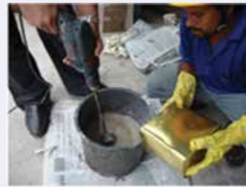
Fig. 5: Mixing of Dr. Fixit Pidipoxy Underlay-SL
