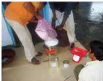
Fig. 17: Mixing of primer Dr. Fixit Pidipoxy EP
