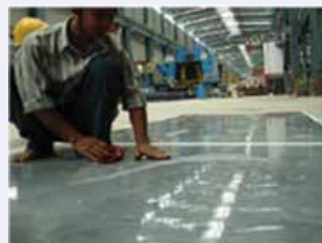
Fig. 7: Application of Dr. Fixit Pidipoxy Underlay-SL
