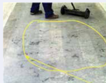
Fig. 15: Scraping of concrete surface and exposing weak floor concrete substrate
