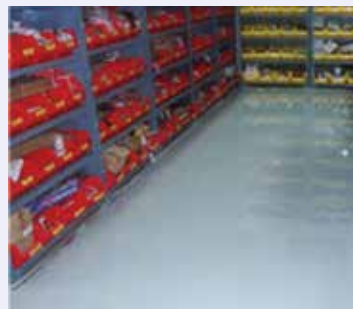
Fig. 22: Floor of Hoovers spares-blast proof machine room after self levelling flooring
