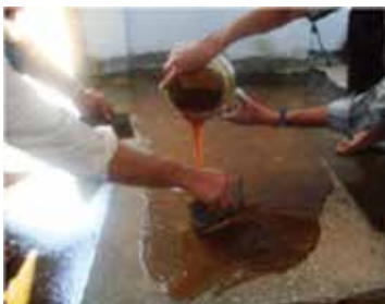
Fig. 19: Mixing of Dr. Fixit Pidipoxy ESL 1000
