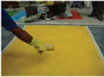
Fig. 9: Application of finished coat with Dr. Fixit Pidipoxy ESL 1000
