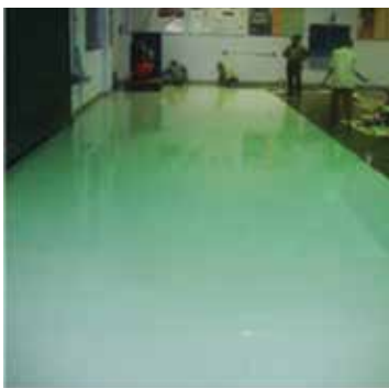
Fig. 26: Workshop Master Bay after self levelling flooring
