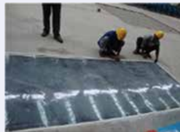
Fig. 6: Application of Dr. Fixit Pidipoxy Underlay-SL
