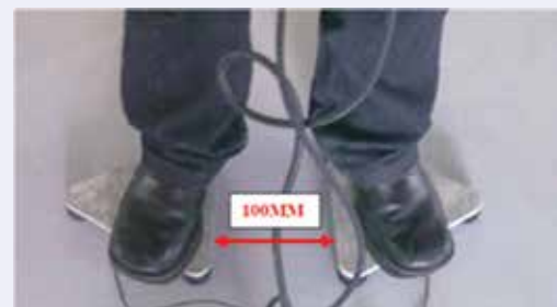
Fig. 28: Checking antistatic property of self-levelling epoxy flooring
