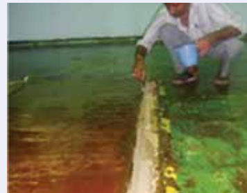
Fig. 14: Sealing moving joints for floor with Dr. Fixit Pidiseal 43
