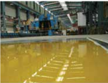
Fig. 10: View of self levelling epoxy industrial flooring after installation
