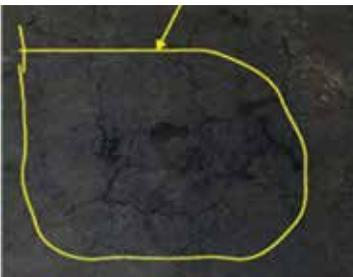
Fig. 12: Cracks in existing floor
