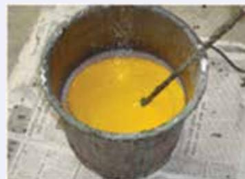
Fig. 8: Mixing of Dr. Fixit Pidipoxy ESL 1000
