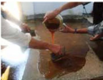
Fig. 19: Mixing of Dr. Fixit Pidipoxy ESL 1000
