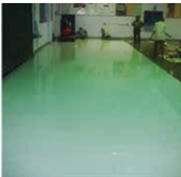
Fig. 26: Workshop Master Bay after self levelling flooring
