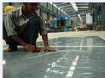
Fig. 7: Application of Dr. Fixit Pidipoxy Underlay-SL
