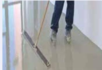
Fig. 2: Spreading self-levelling cementitious flooring product
