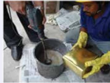
Fig. 5: Mixing of Dr. Fixit Pidipoxy Underlay-SL
