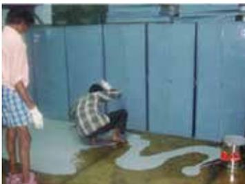
Fig. 18: Application of Dr. Fixit Pidipoxy EP
