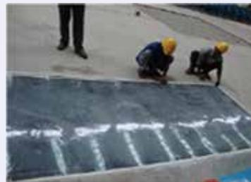
Fig. 6: Application of Dr. Fixit Pidipoxy Underlay-SL
