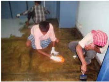
Fig. 16: Priming of floor surface
