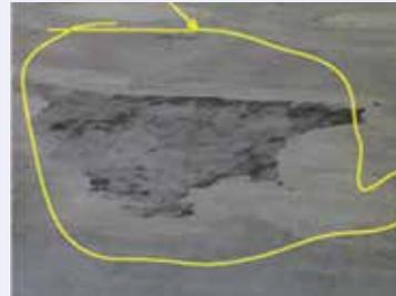
Fig. 13: Debonding of floor surfaces due to wear and tear
