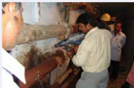
Fig. 5: Electric drill - Heavy duty - power output - 1050 watts and drill speed - 350-600 rpm with variable speed control
