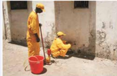
**Fig. 14:** Injection with silicate based injection grouts for raising dampness in masonry wall
