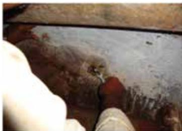
Fig. 8: Fixing the packers in drilled holes
