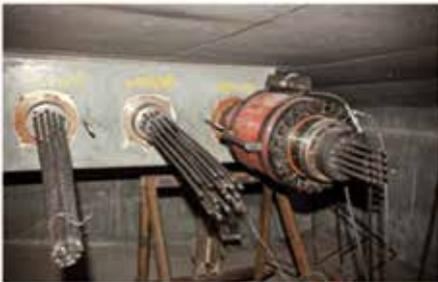
Fig. 18: View of post tension tendon duct for grouting
