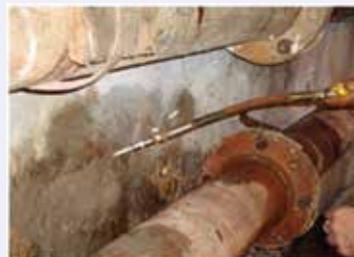
Fig. 11: Grouting hose pipe, Ball valve and Injection packer fixed with epoxy putty and PU grouting in action in a dam project
