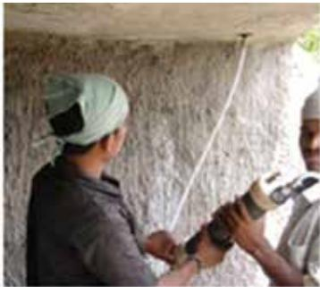
**Fig. 12:** Grouting in action with a hand pump in a deck slab of highway culvert with epoxy injection grouts
