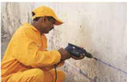
**Fig. 13:** Drilling the hole by a drill bit at 45° downward
