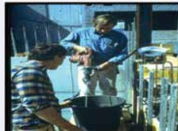
Fig. 9: Mixing paddle - Should be capable of producing high shear during mixing of cementitious grouts
