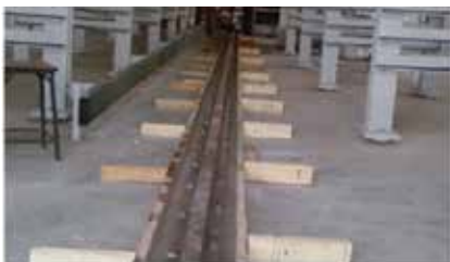
Fig. 1: View of rail 1 and base plates of steel columns
