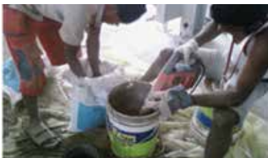
Fig. 5: Mechanical mixing of grout material in a container
