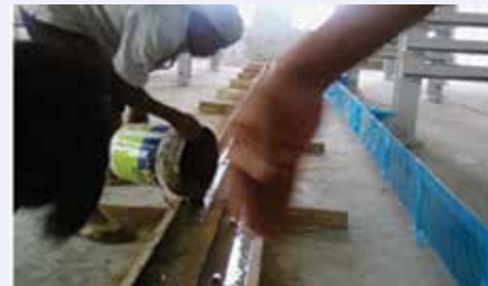
Fig. 6: Pouring of grouts for fixing rail 1
