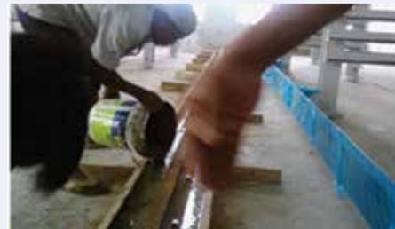
Fig. 6: Pouring of grouts for fixing rail 1
