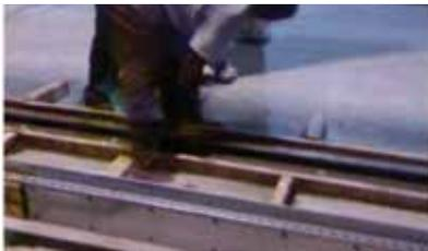
Fig. 3: Removing dust by air compressor
