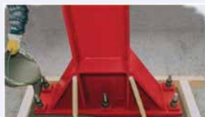
**Fig. 16:** Grouting below a column base plate
