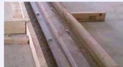
Fig. 2: View of form work and the rail being placed firmly before grouting
