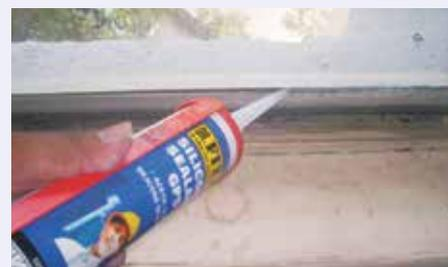
Fig. 7: Silicone sealant between frame and masonry
