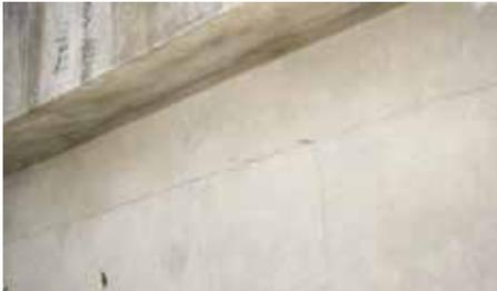
Fig. 2: Cracks are routed cleaned and prepared
