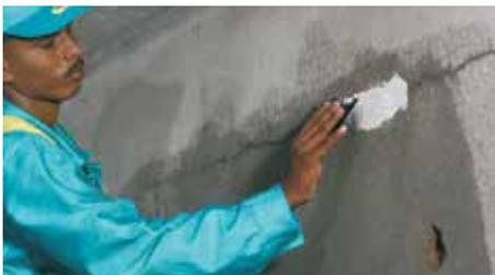
Fig. 3: Crack filling with polymeric repair material
