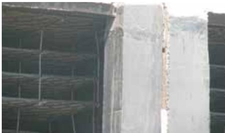
Fig. 6: PU sealant at construction joint
