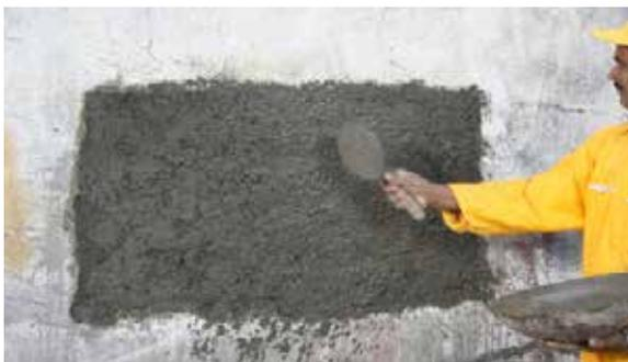
Fig. iii: Application of polymer mortar
