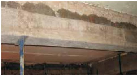
Fig. 4 iv : Repair done by micro concrete
