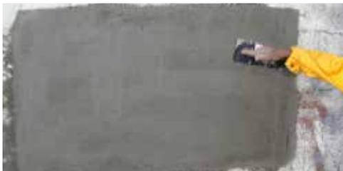
Fig. 1 v: Finishing with a trowel
