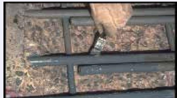
Fig. 1 ii: Priming the steel with zinc epoxy primer after rust removal
