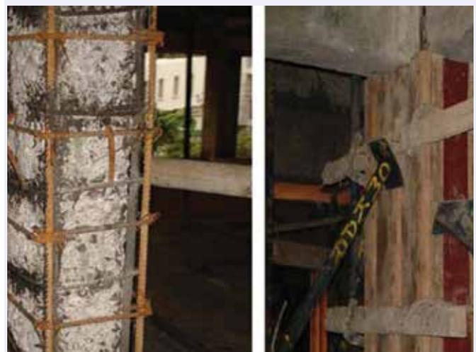
Fig. 4 ii : Micro concrete for repair of a congested beam
