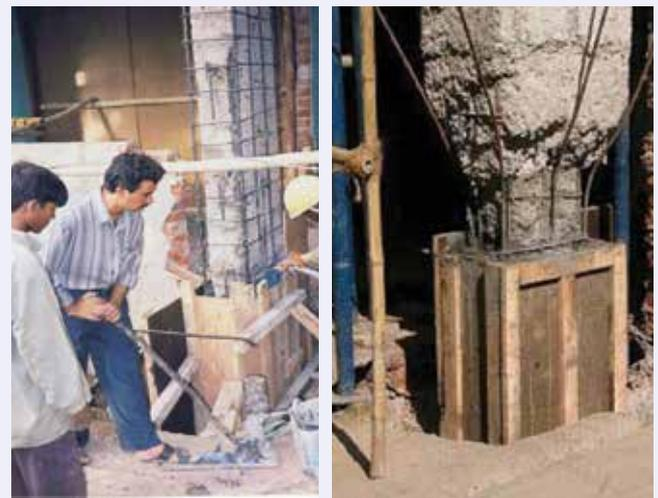
Fig. 4 i : Micro concrete for repair of a congested beam
