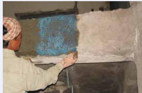
Fig. 2ii : Bonding agent applied for finishes
