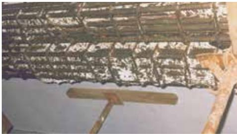
Fig. 4 iii : Micro concrete for repair of a congested beam
