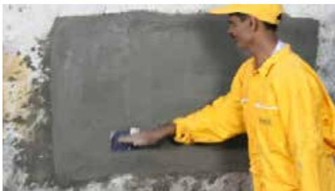
Fig. 1 iv: Striking of excess material
