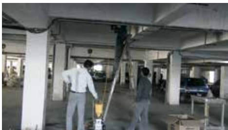
Fig. 2 d: Injection in progress
