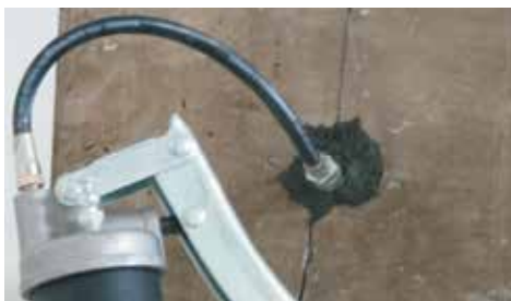
Fig. 2 c: Fixing the hose into the packer and start pumping
