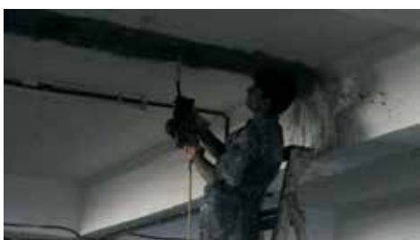
Fig. 2 e: Injection in underside
